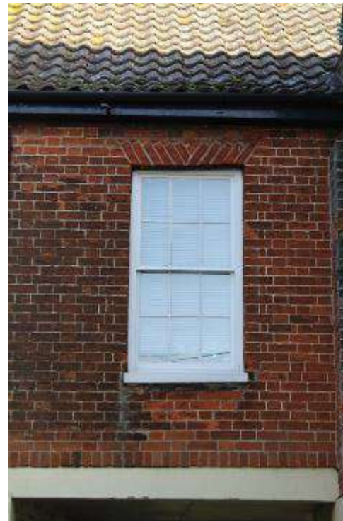
Figure 64 Examples of 'V' shaped red brick lintels
